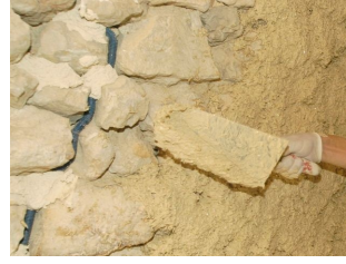
(b) Coating with a trowel ( 800 - 900\ \text{kg.m}^{-3} ).
